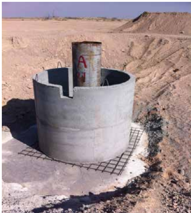
Fig 8.2 – Cellar Preparation
