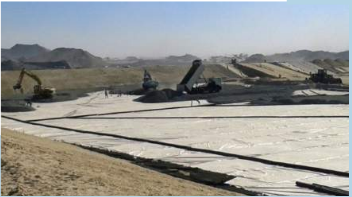
Figure 5.12 South-East Kuwait Landfill- laying down of Geotextile & Leachate Piping Network
