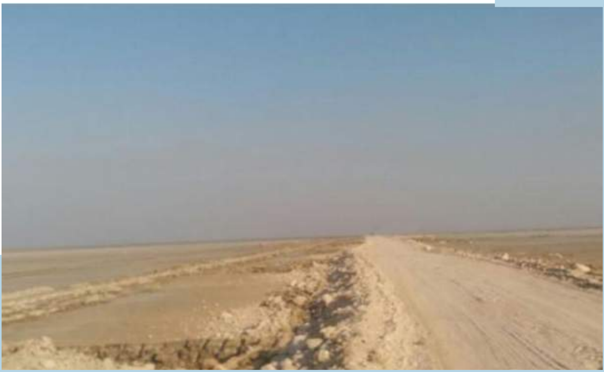
Figure 5.46 Coastal trench after excavation in NK area
