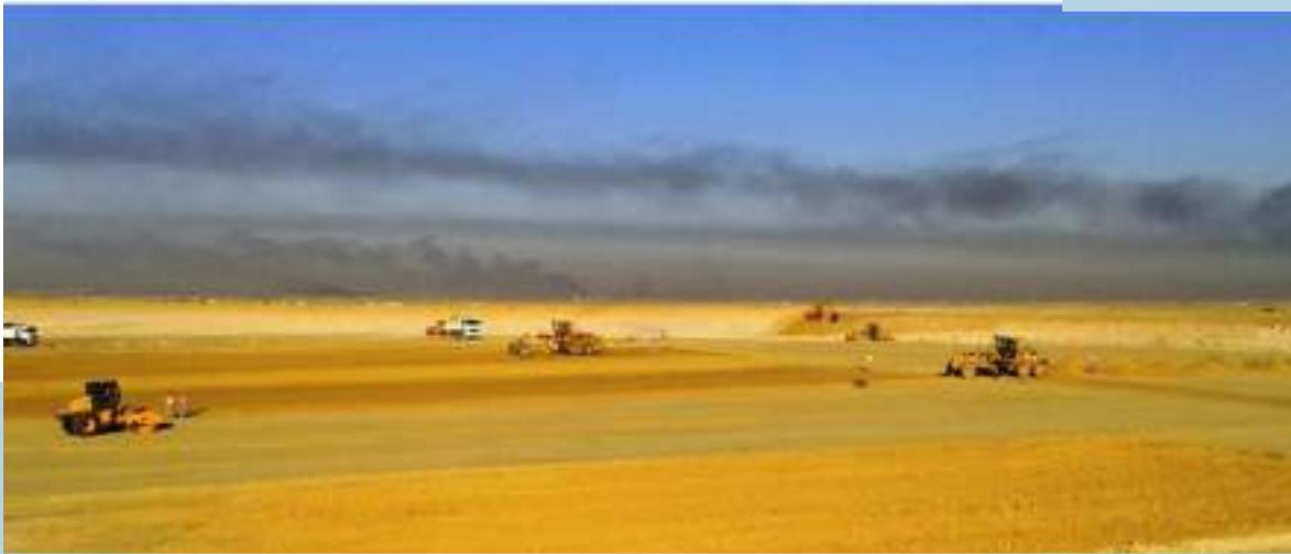
Figure 5.8 South-East Kuwait Landfill-Laying down of Leachate Piping Network
