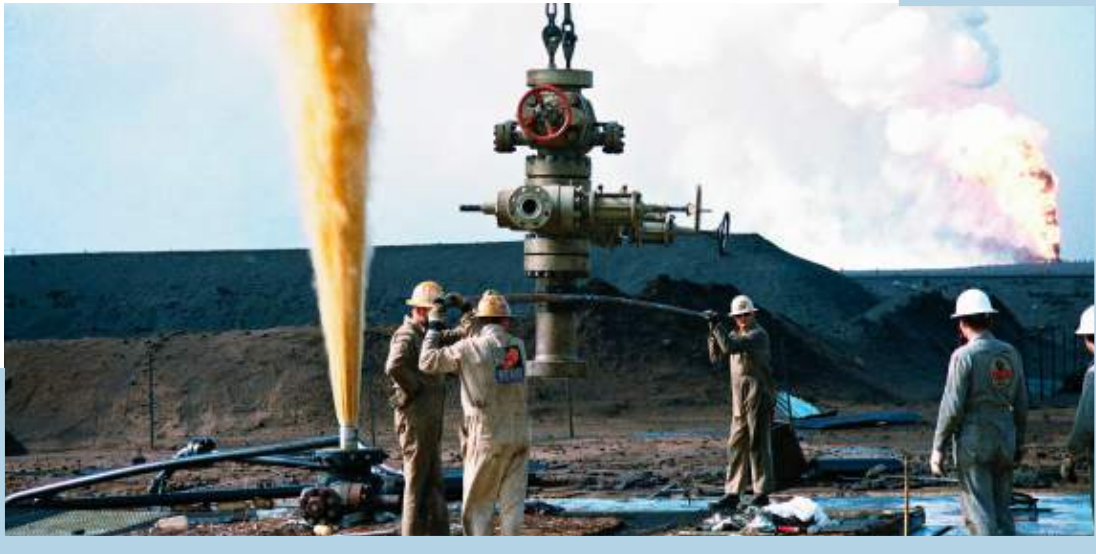
Figure 2.1 Bursted oil wells
