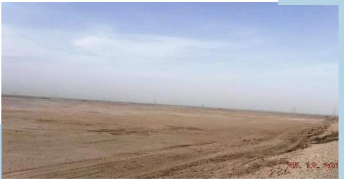
Figure 5.31 Wet Oil Lake after excavation in NK area
