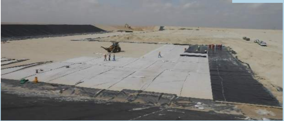
Figure 5.14 North-Kuwait Landfill- Drainage Geotextile/Geomembrane Placement Bottom Base
