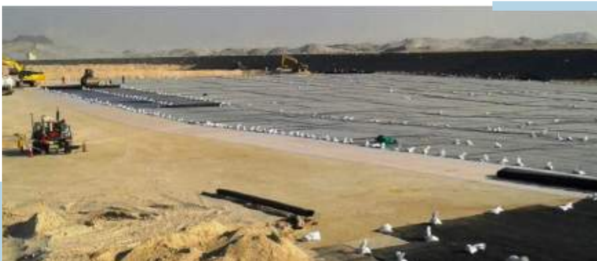
Figure 5.5 Landfill Base Liner System - Materials
