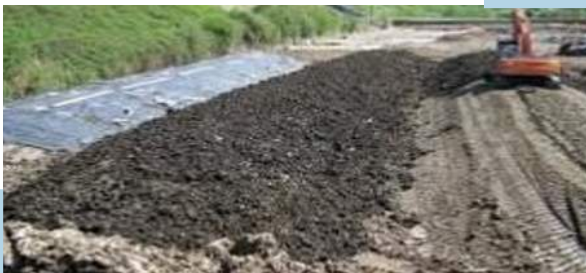
Figure 6.29.2 Landfarming Process demonstration
