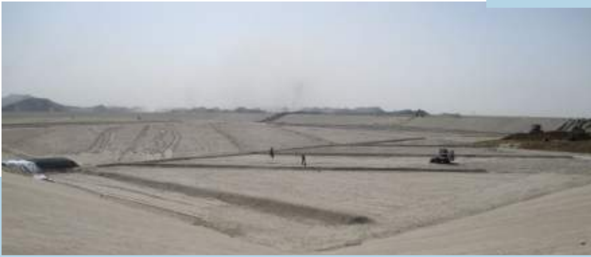
Figure 5.8 South-East Kuwait Landfill-Laying down of Leachate Piping Network
