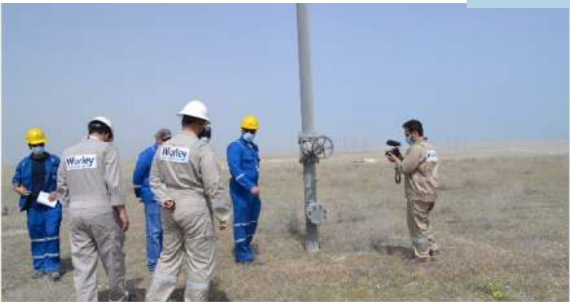
Figure 5.17 North-Kuwait Landfill- Passive Gas Venting Well
