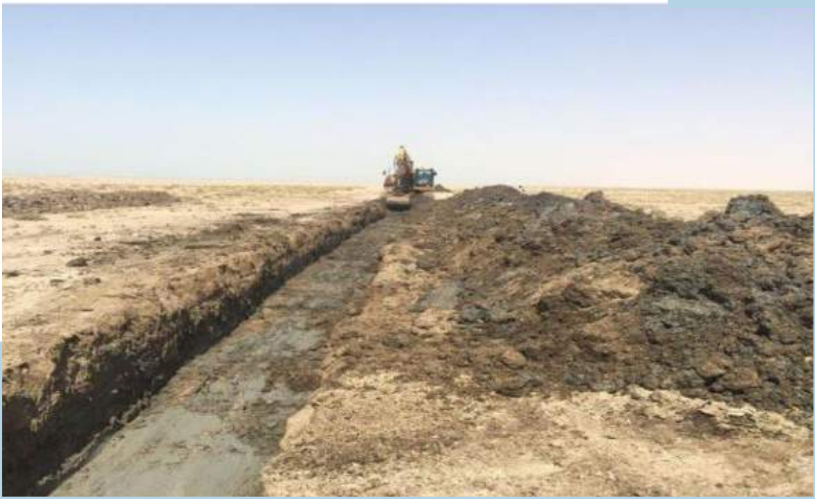
Figure 5.45 Coastal trench during excavation in NK area
