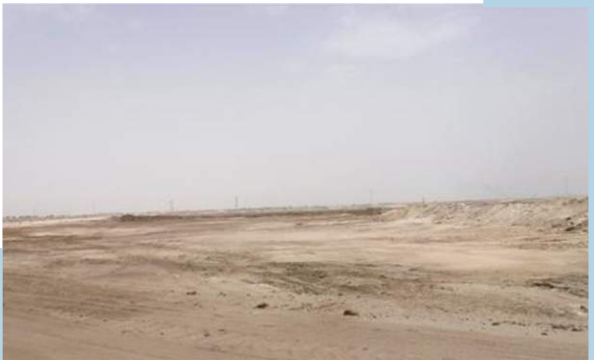
Figure 5.44 Contaminated Soil Piles after excavation in SEK area
