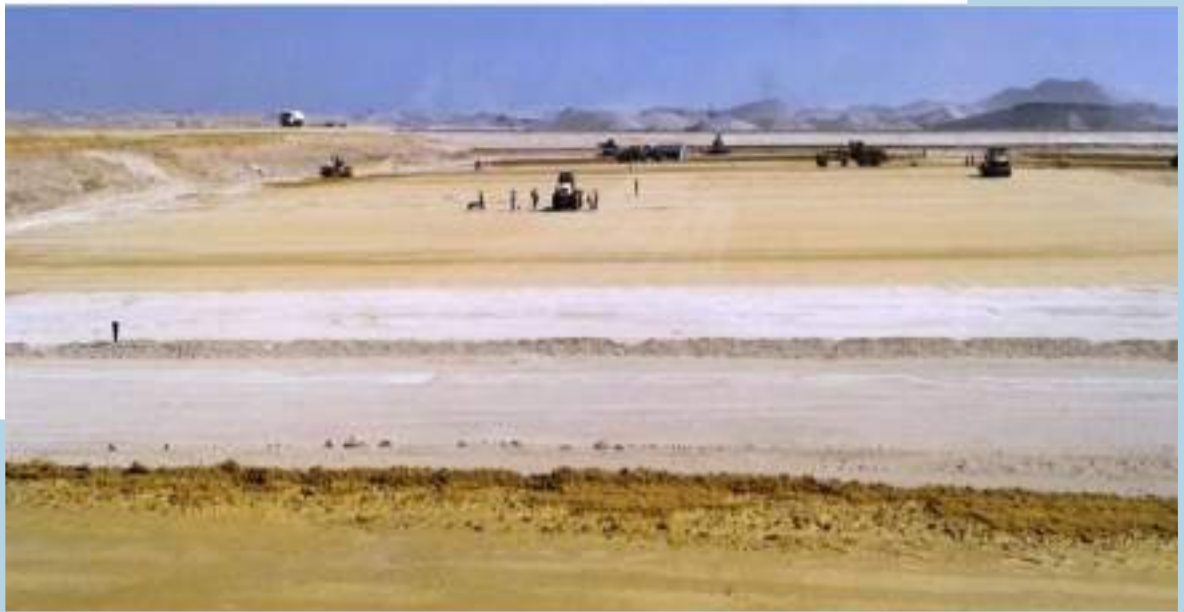
Figure 5 3 South-East Kuwait Landfill-Grading and Compaction
