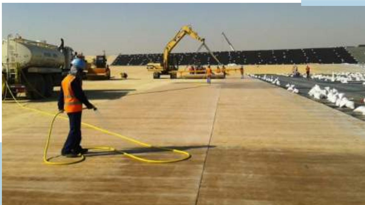
Figure 5.13 South-East Kuwait Landfill Laying Down of Geo Synthetic clay liner
