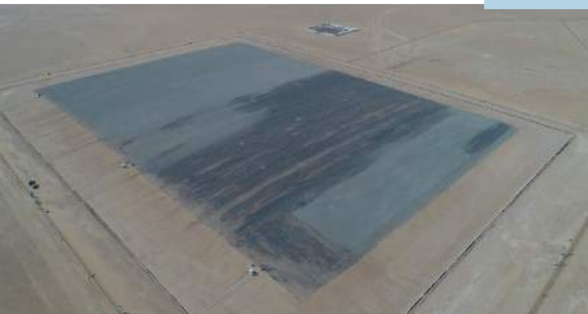
Figure 5.2 North Kuwait Capped Landfill- Top View
