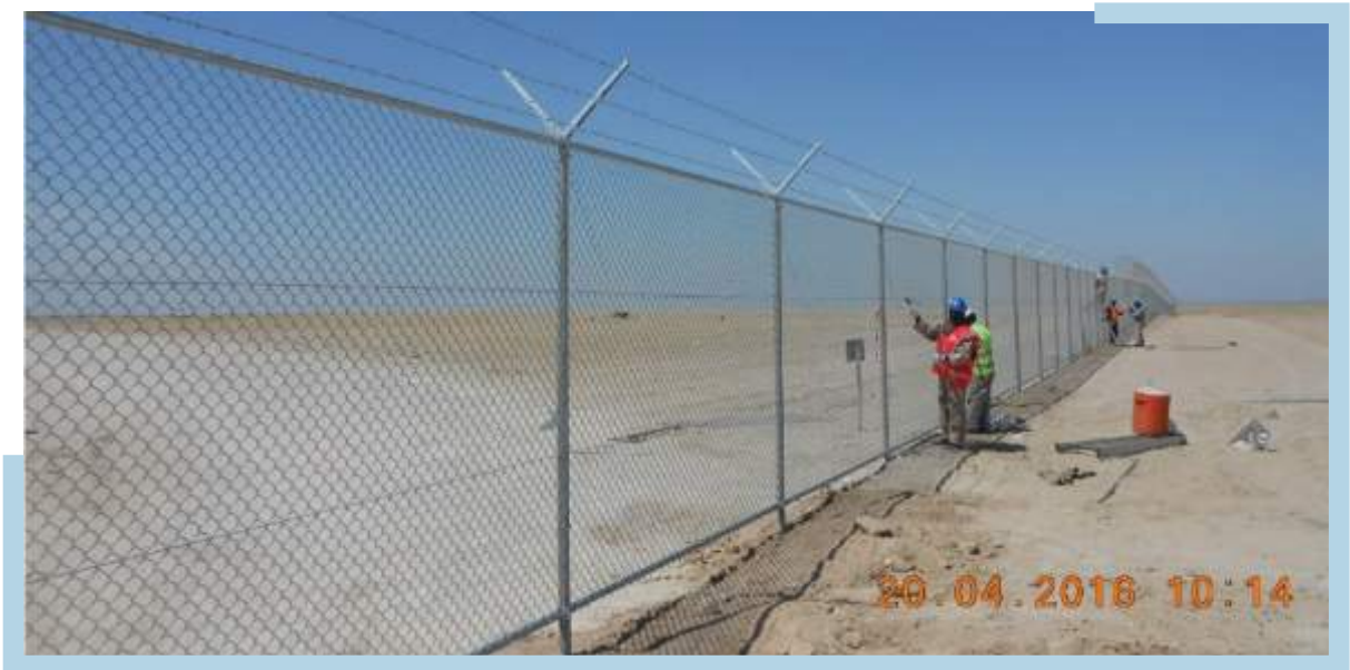
Figure 5.18 South East-Kuwait Landfill- Fence Construction
