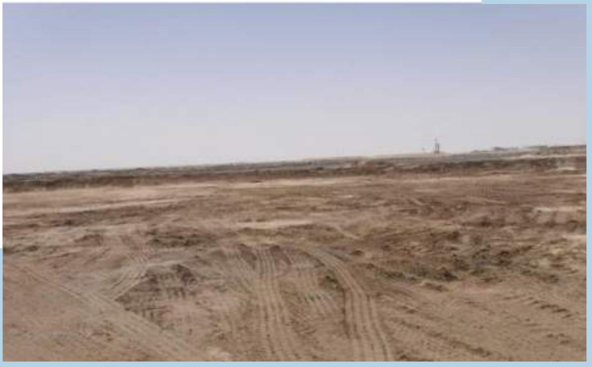
Figure 5.35. Contaminated Soil Piles after excavation in NK area
