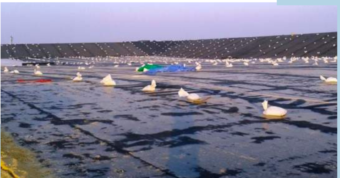
Figure 5.11 South-East Kuwait Landfill- Laying down of HDPE Geomembrane
