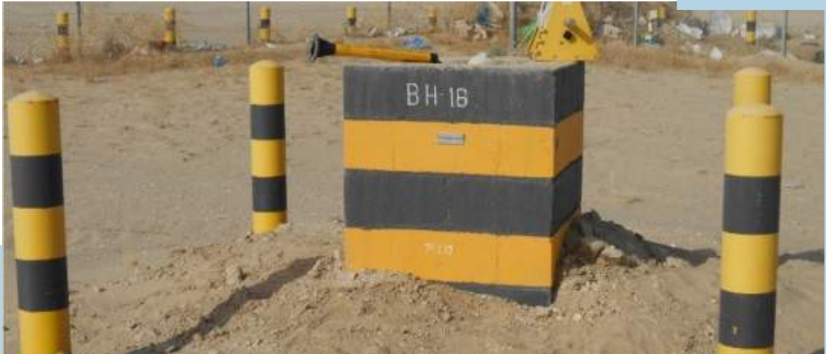
Figure 5.20 South East-Kuwait Landfill- Groundwater Monitoring Well
