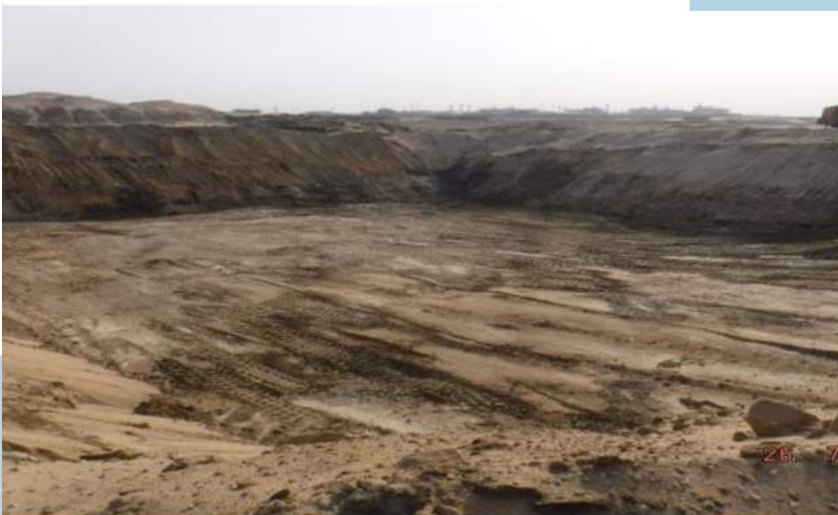
Figure 5.42 Wellhead pits after excavation in SEK area
