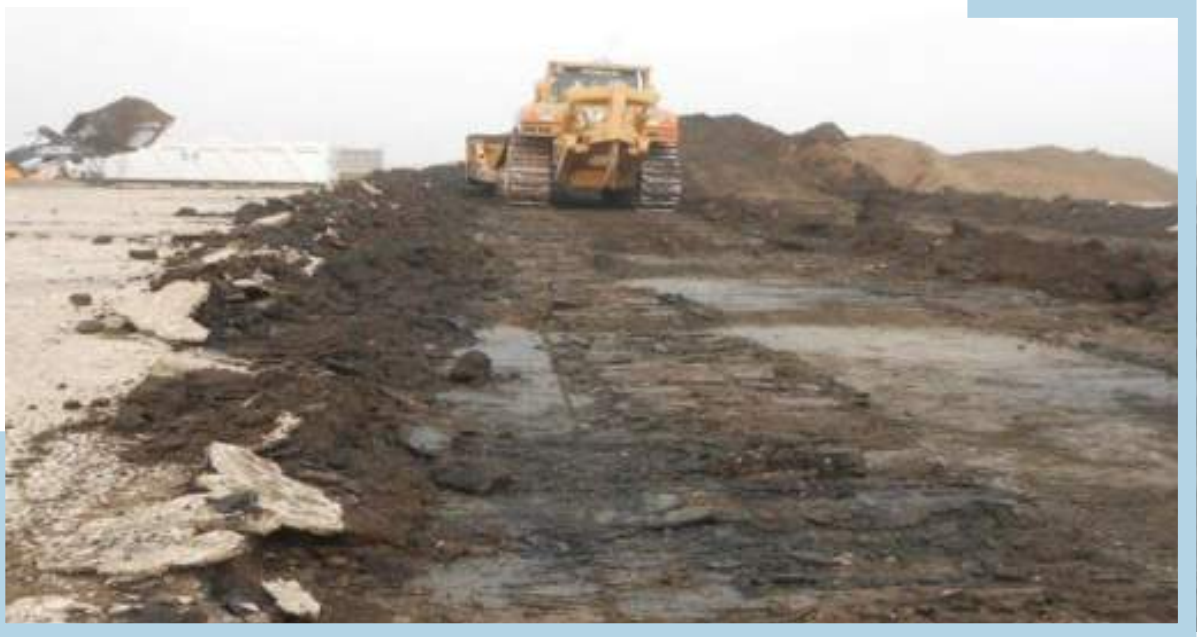
Figure 5.32 Dry Oil Lake during excavation in NK area
