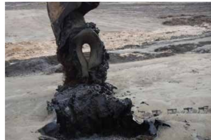
Figure 34. Excavation of oil contaminated soil
