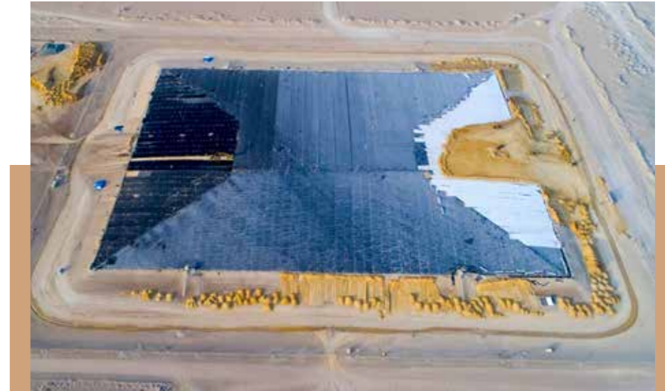
Figure 17. Construction of landfill in SK.
