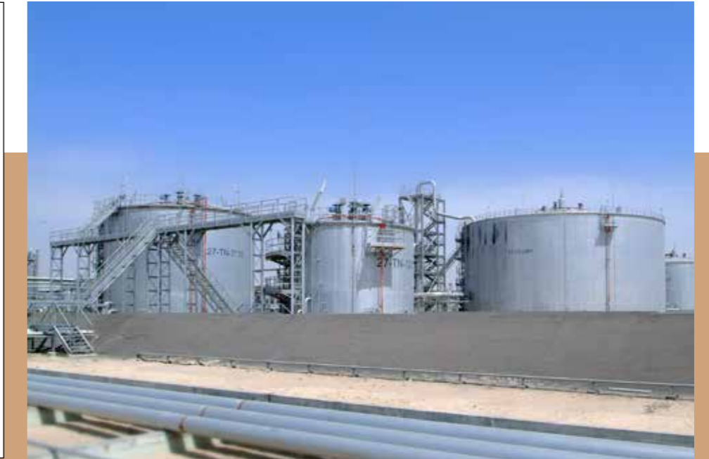
Figure 22. Recovered oil in storage tank.
