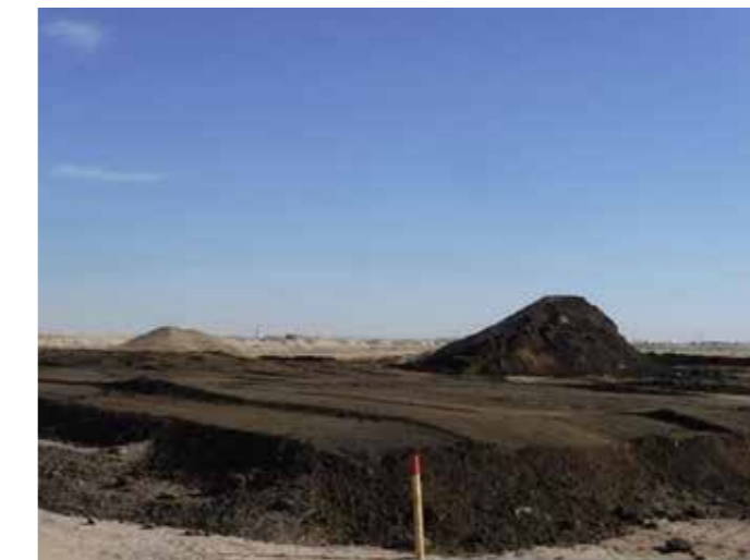
Figure 28. Oil contaminated pile before remediation.
