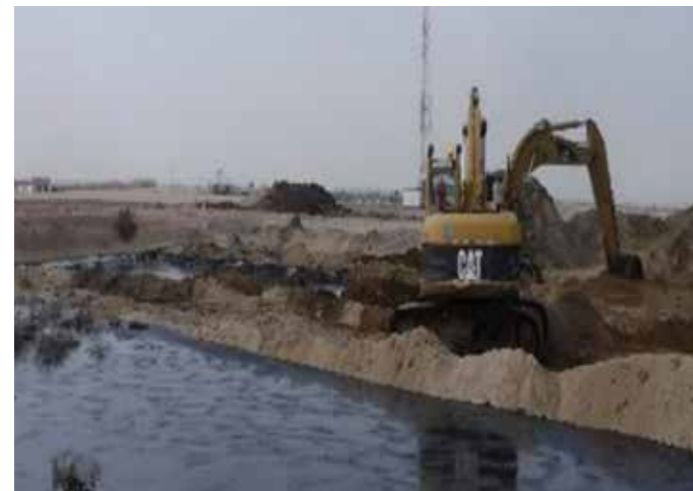
Figure 32. Wellhead pit before remediation
