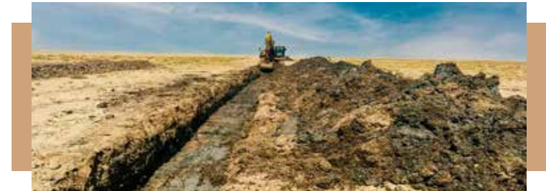
Figure 5. Coastal oil trench in Al-Subbiyah, Kuwait
