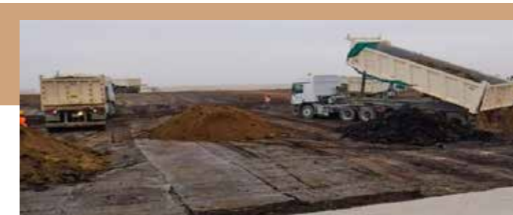
Figure 16. Filling oil sludge after lining SK.
