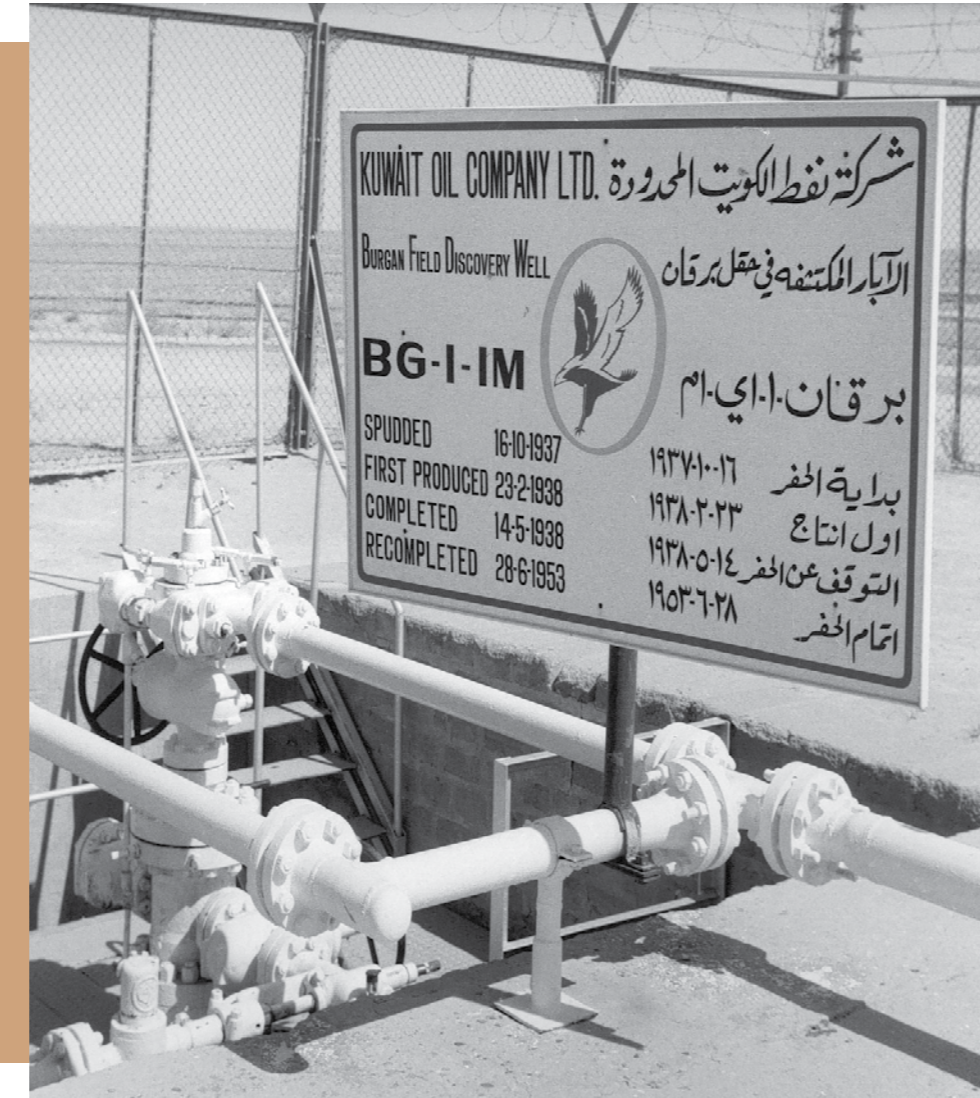
Figure 1. The oldest oil well at Greater Burgan installed in 1938 (numbered BG-1 IM) [1]
