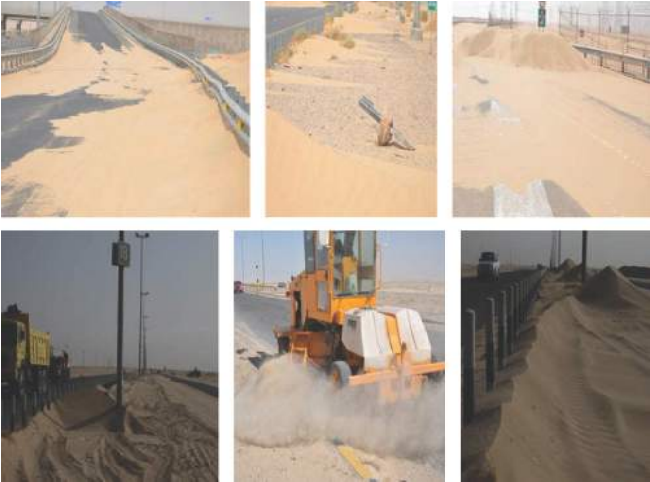
Figure 2.8 Consequences of soil erosion by wind (top is Sabiya Road; bottom is Wafra, Mina Abdallah Road) (June 2015) 2
