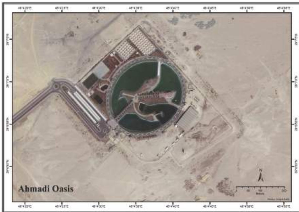
Figure 6.4 Aerial view of the Ahmadi Oasis
