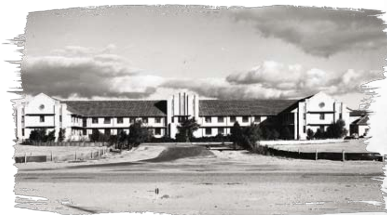
KOC Main Office
