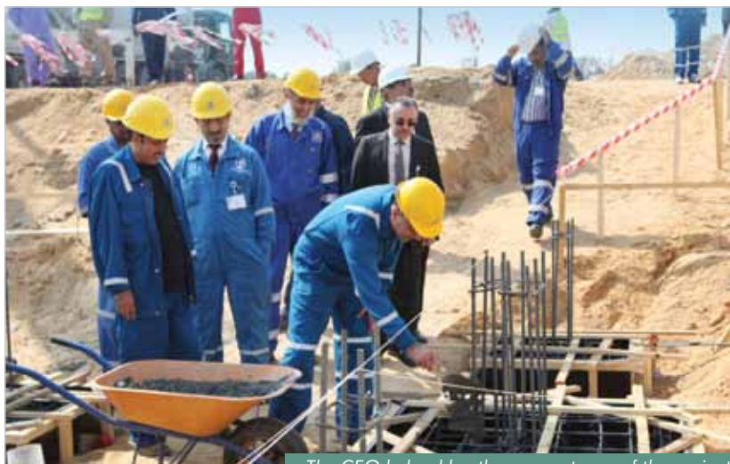
The CEO helped lay the cornerstones of the project.
